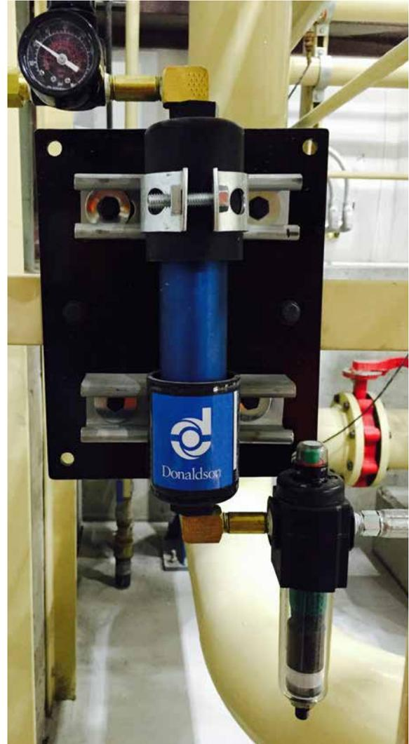
\*The Reservoir Air Dryer is not recommended for use on gasoline holding tanks, or for the head space of any flammable liquid (Flash Point below 100°F / 38°C)
